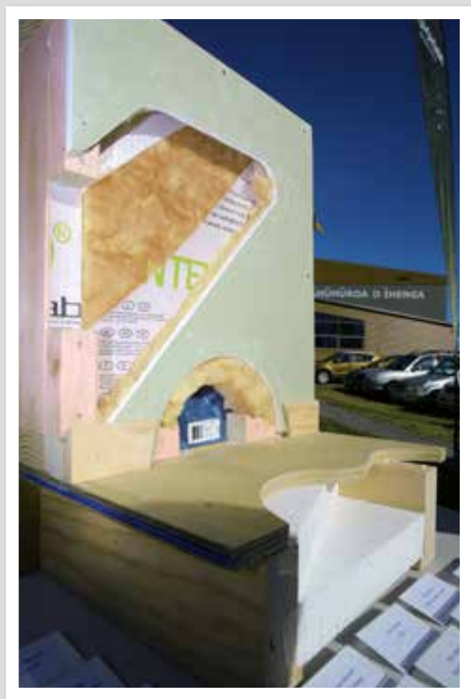
CROSS SECTION OF THE INSULATION SYSTEM IN THE LATEST CHARITY HOUSE BUILT
